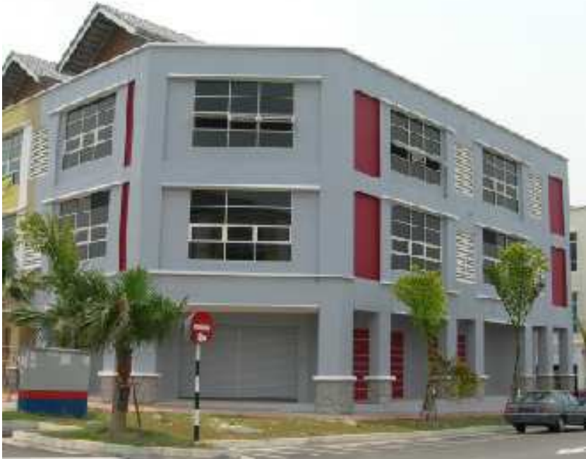
Front view of the NiSCell; 3500Sq. ft of Class 10K space will house 4 cGMP clean rooms
